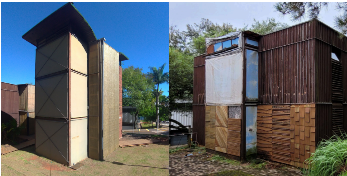
Figure 1: Experimental Housing Units 001 (Left - East view) and 002 (Right - West view)
