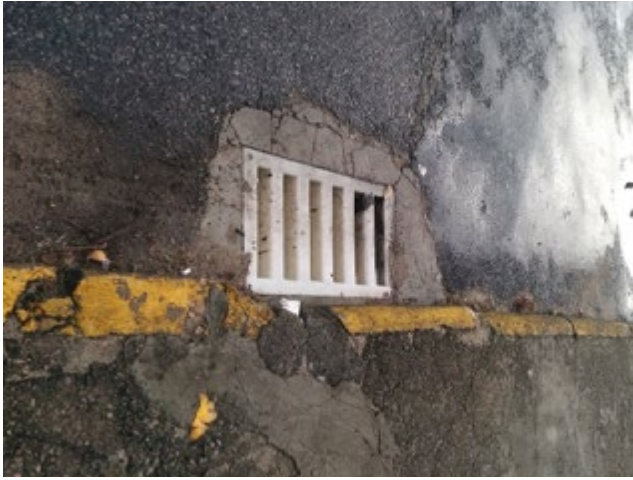
Figure 9 – Drain grate model showing positive affordance for rainwater collection but no negative affordance for trapping bicycle wheels. Rua Altamiro Barcelos Dutra, Florianópolis, Brazil Source: Authors.
