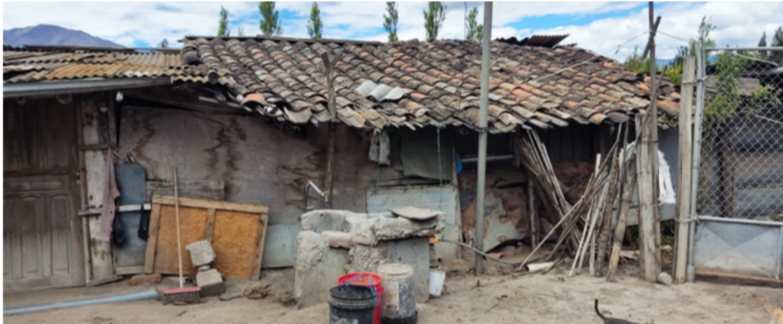
Figura 3 – Building with a construction technique similar to wattle and daub observed in Salinas
