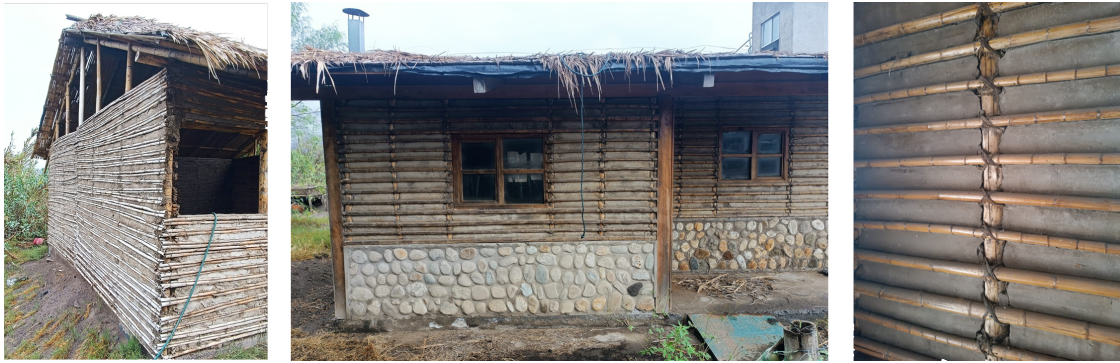
Figura 4 – Wattle-and-daub adapted buildings of the Museo de la Sal in Salinas
