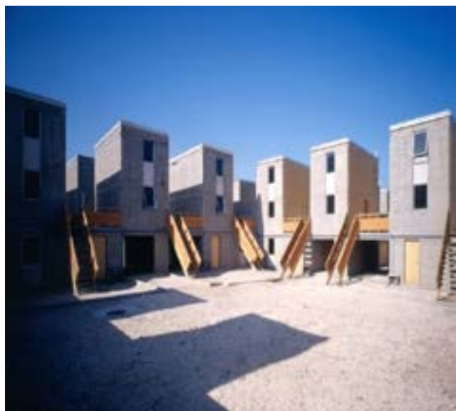
Figure 3 : Quinta Monroy housing complex, Chile.
