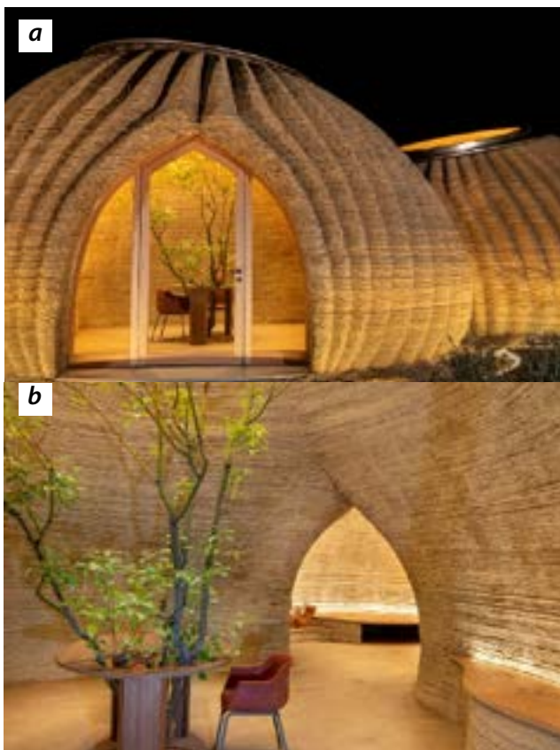
Figure 4: (a) TECLA house finished externally; (b) internally Source: (PINTOS, 2021)
