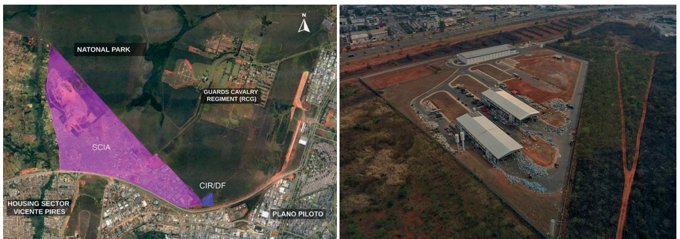
Figure 01: Location map and aerial view of the CIR/DF study area. Source: adapted from Google Maps and LaSUS/UnB, 2023.
