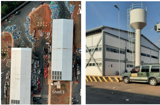
Figure 02: Images of the sheds and facade of shed 1. Source: LaSUS/UnB and Authors (2023).
