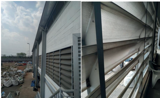
Figure 03: Facade with openings in the shed. Source: LaSUS/UnB and Authors (2023).
