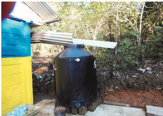
Figure 05 – The autonomous design of Catalina - Water collection system made by Catalina. Source: Catalina Santiz (2019)
